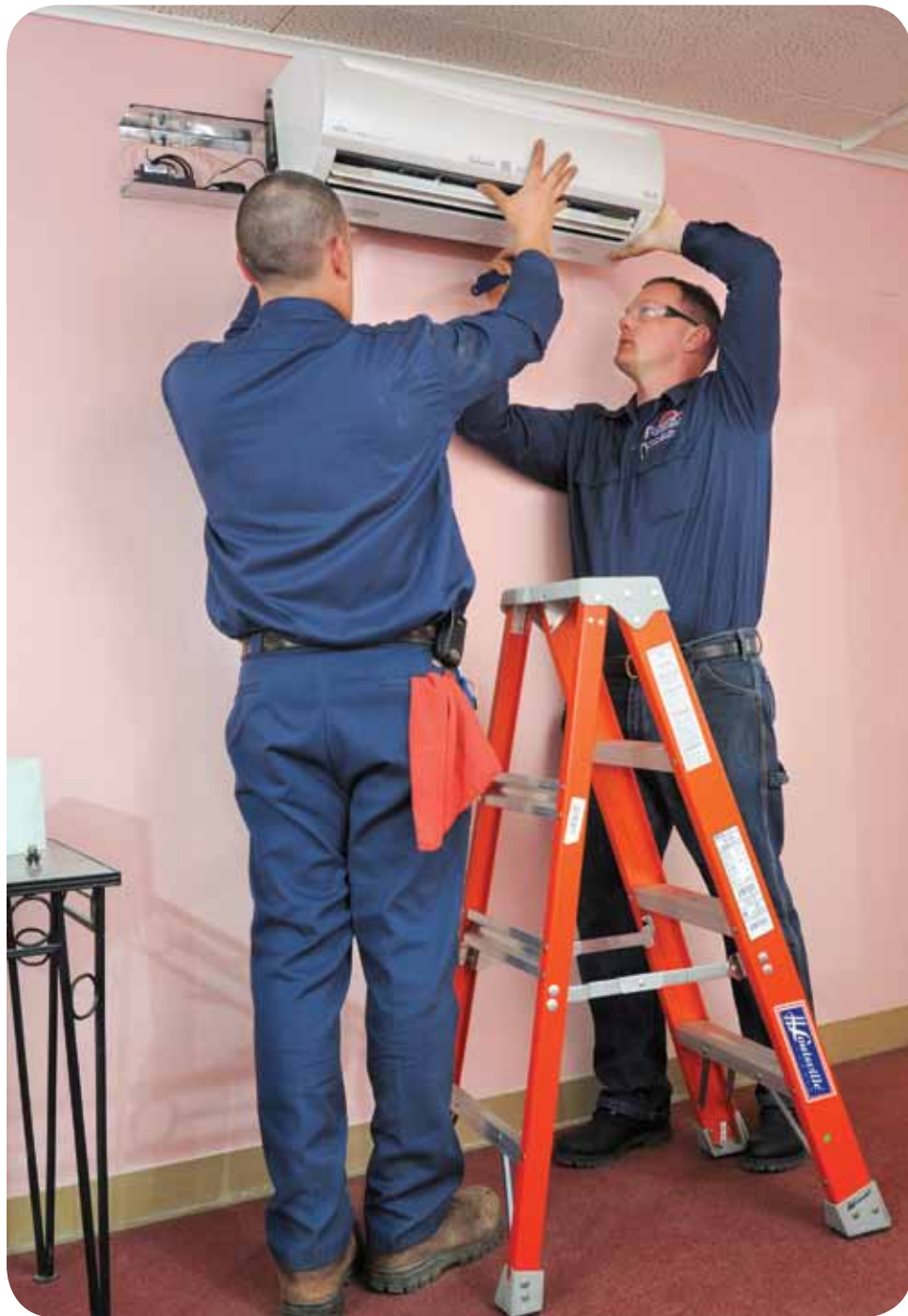
Technicians Carl Einsig and Jamie Schrum handle the indoor evaporator section of the new ductless units installed at the Heidelberg United Church of Christ in York, Pa.
