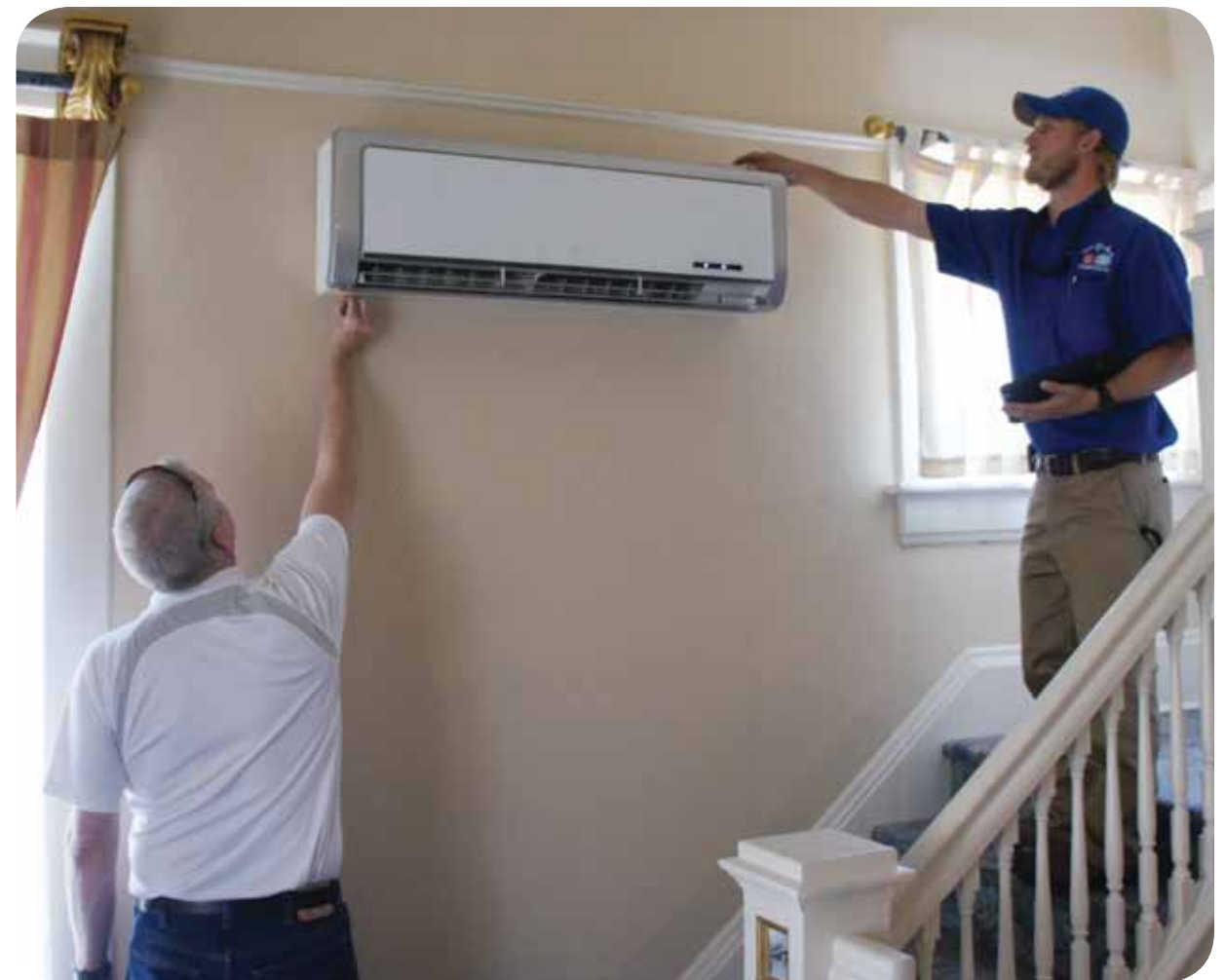
Contractors with Champion AC, San Antonio, carefully set a newly installed wall-mounted ductless air conditioner into place.
